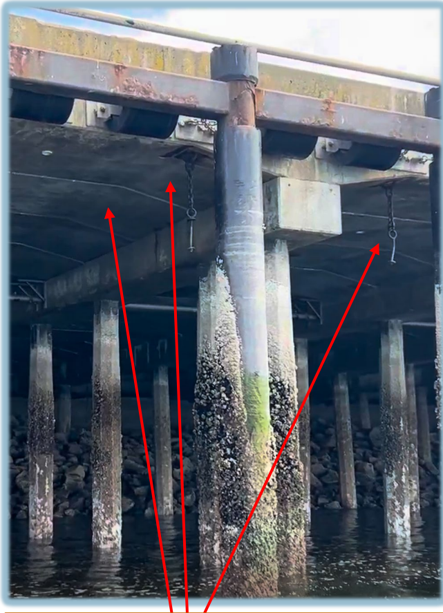
Precast concrete deck panels from below Pier 91
