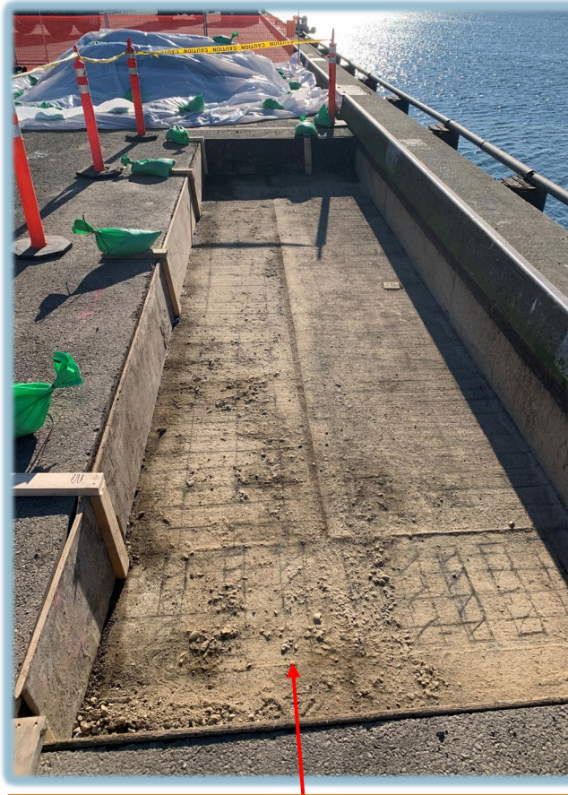
Precast concrete deck panels from top of Pier 91
