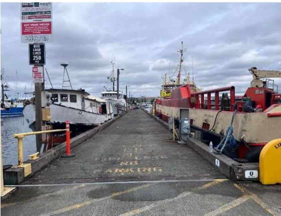
NW Pier2 North
