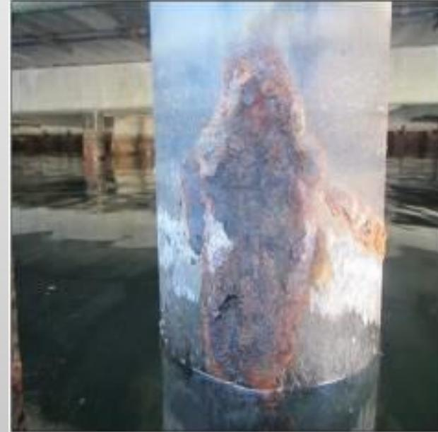
*The steel piles supporting FiT Docks 3, 4, and 5 were installed in the early 1980s. The piling consists of thin steel hollow pipes filled with unreinforced concrete. The pile system provided reliable service for the past 35 years, but corrosion is manifesting within the splash zones and near the mud line of some piling, compromising the integrity of the system and requiring the prevention of future corrosion.*
