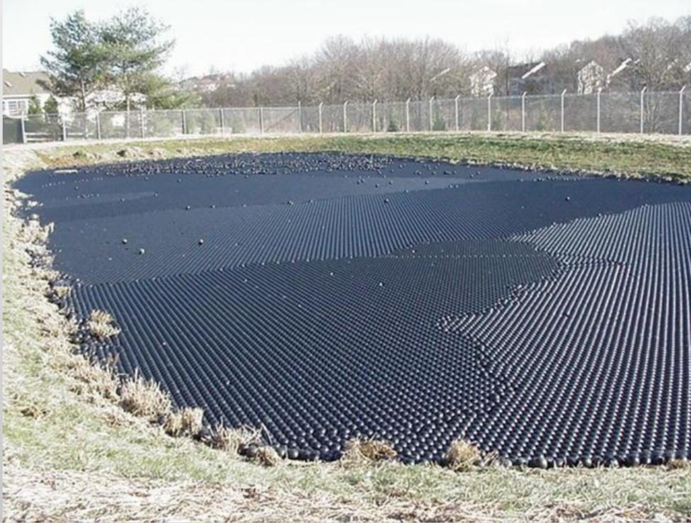
Floating balls are a long-term, easy to install, low maintenance option
